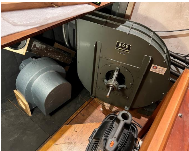
Figure 1 Main chamber New blower left; original 'BOB' (British Organ Builders) right
