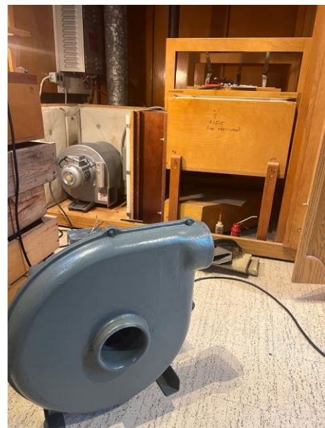
Figure 2 New gallery blower in the silencing box; original blower forefront
