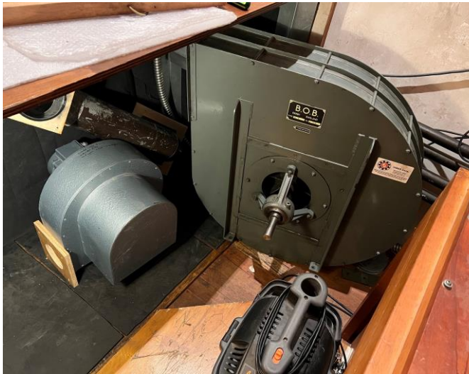
Figure 1 Main chamber New blower left; original 'BOB' (British Organ Builders) right
